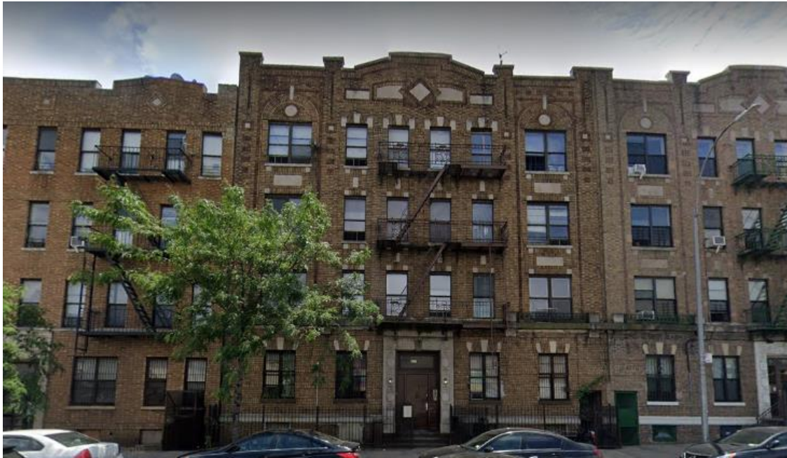
The exterior of 2178 Atlantic Avenue.
